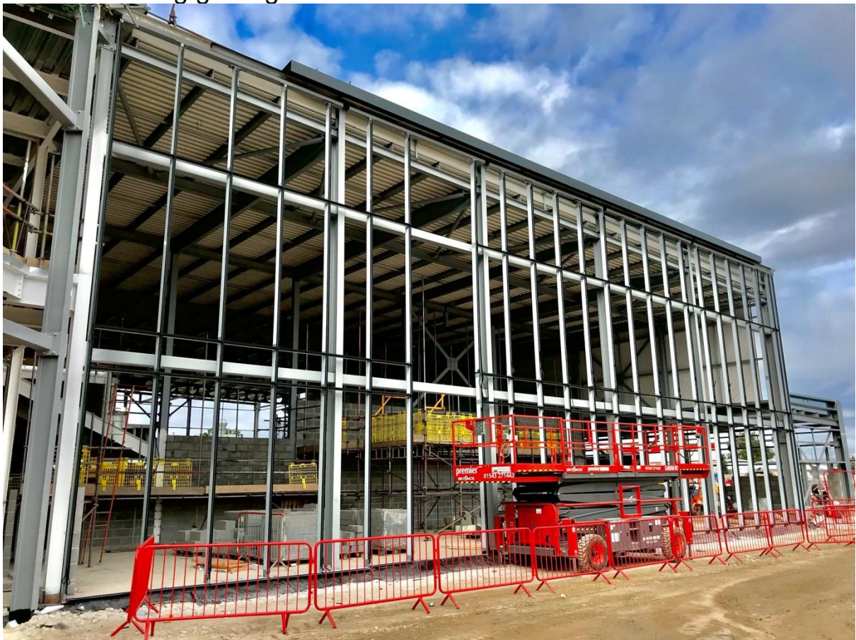
Leisure Building glazing frame installation:
